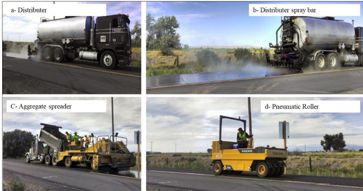
Figure 1-4 Chip seal construction sequence (Photo credit Paul Ledtje)
